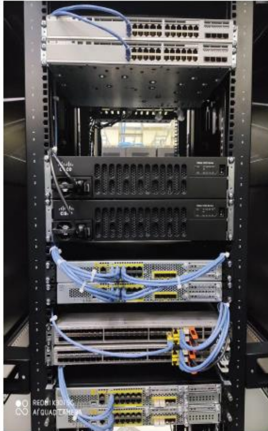
Site Photo (Front View)
